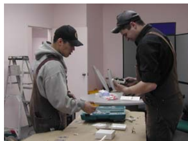
Bobby Makpah and Steve Fitzpatrick working on the electrical system for the office.
